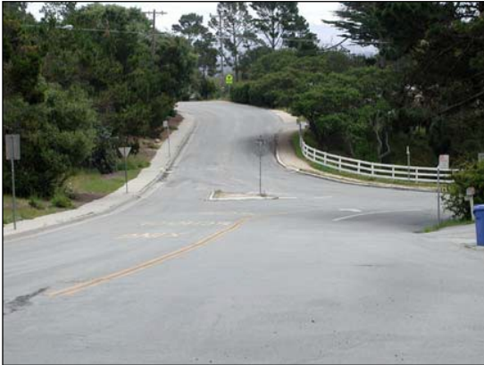
Figure 7: Mar Vista Drive Toward Soledad Drive
