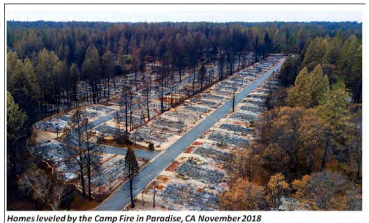
Homes leveled by the Camp Fire in Paradise, CA November 2018
