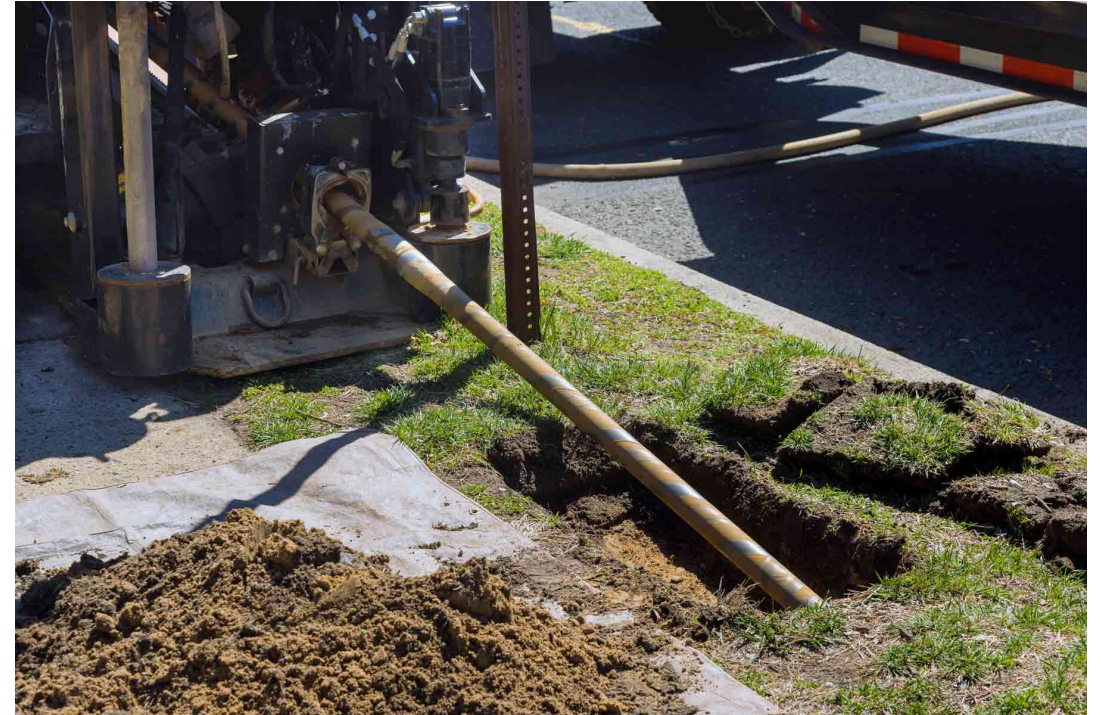
Directional Boring allows undergrounding without digging trenches
